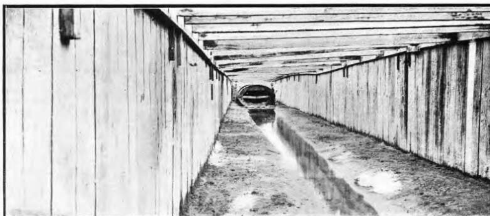
6 ft. diameter Storm Water Concrete Drain, in course of construction.
