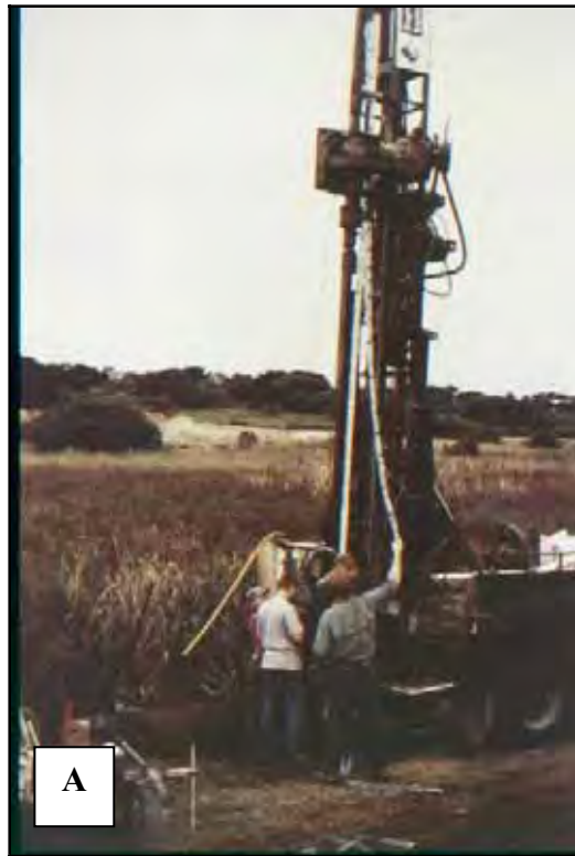
Figure 5.4 Bundled piezometer installation; (a) installing piezometer sections through hollow-stem augers, and (b) augers ready for retraction.
